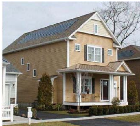
Reynolds Farm is the first community in Rhode Island to feature DOW Powerhouse Solar roof shingles
